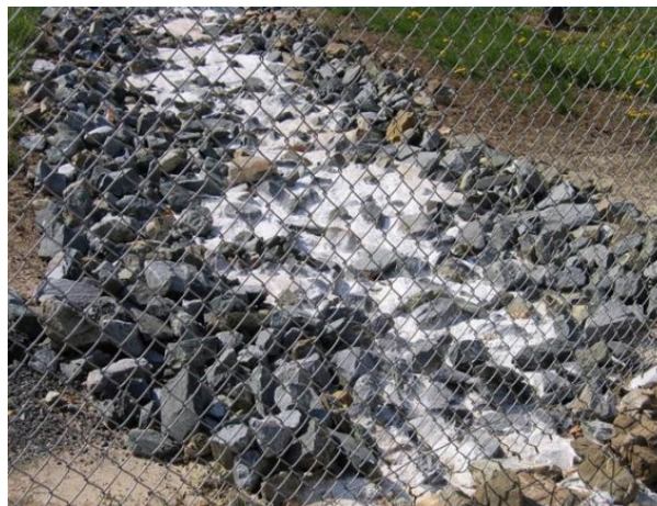
Figure 48. Stormwater swale affected by salt washoff (MDOT 2022).
